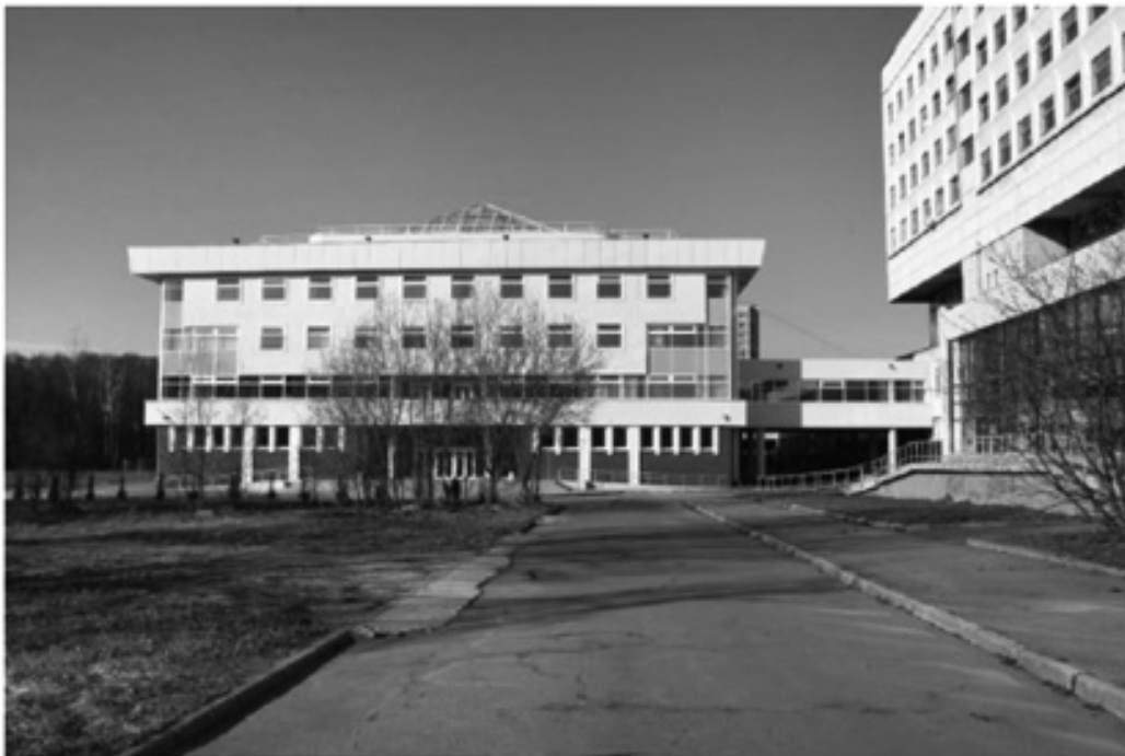
Figure.1 Educational Laboratory Building, equipped with energy-efficient automated control system.
